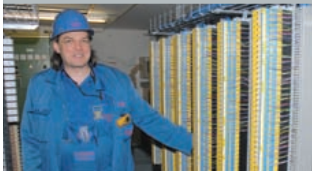
IM34 compact temperature measuring transducers replace old 19-inch cards at BP Lingen Page 36
