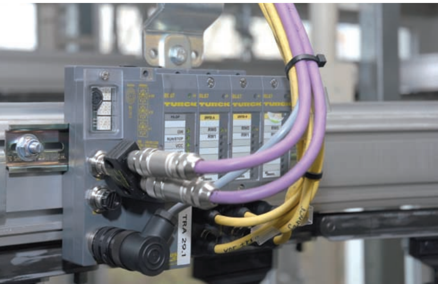
Seven I/O stations with Profibus interface cover a total of 28 read/write heads, which read the UID of the data carriers
